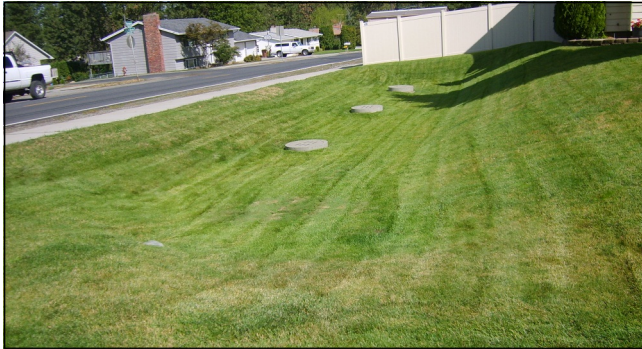
This vegetated swale requires a Tier I inspection
