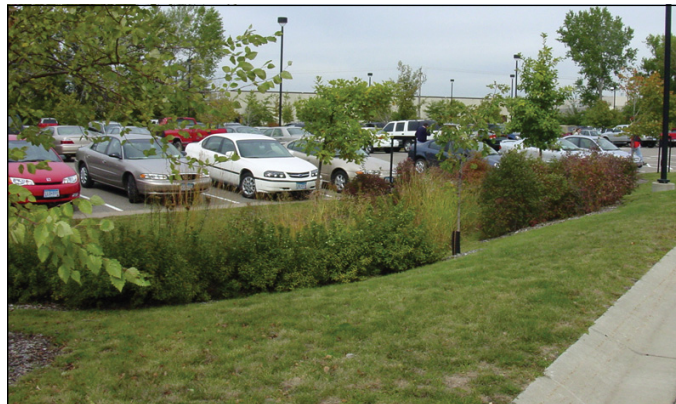
This bioretention cell requires a Tier III inspection
