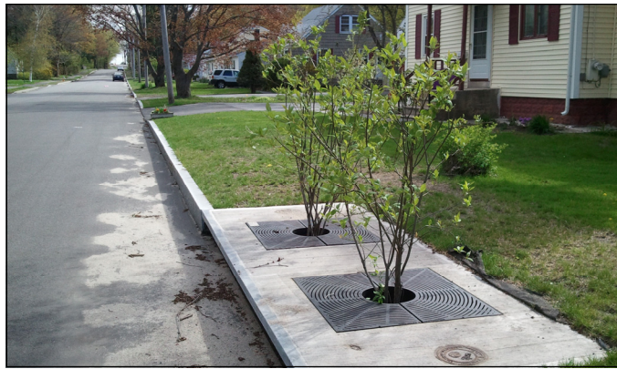
This tree box filter requires a Tier II inspection
