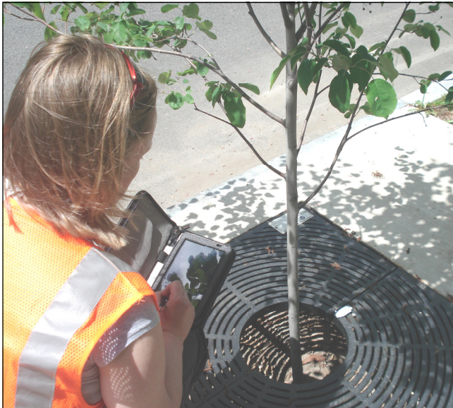
CCSWCD staff inspects a tree box filter
